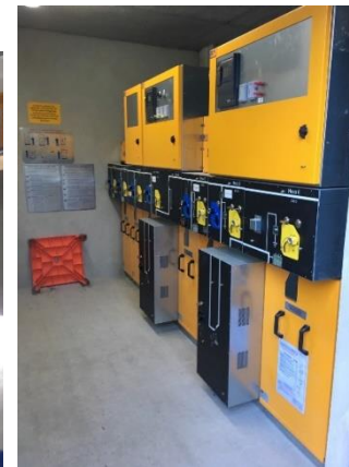
Cellules MT Cellules BT Protections
